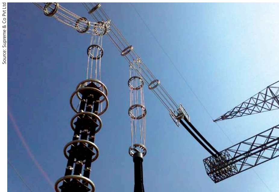
1200 kV power transmission system with improved insulator and conductor fittings
